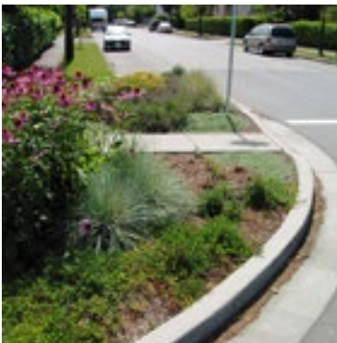
Landscaped bulb outs can be utilized to tighten a curb and provide shorter crossing distances.
