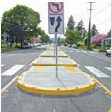
Lanes can be narrowed and traffic slowed by installing pedestrian islands, bike lanes, and on-street parking.
